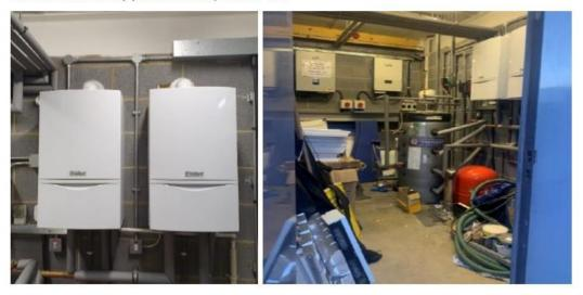
The requirement is that an additional cascade control system is installed to interlink the boilers. When boilers are linked, they communicate with each other and work in tandem to increase or decrease heat output as and when needed.
